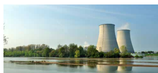
Perimeter monitoring for nuclear facilities
